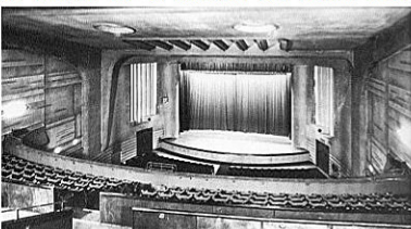
The auditorium - repairs to the ceiling are clearly visible
